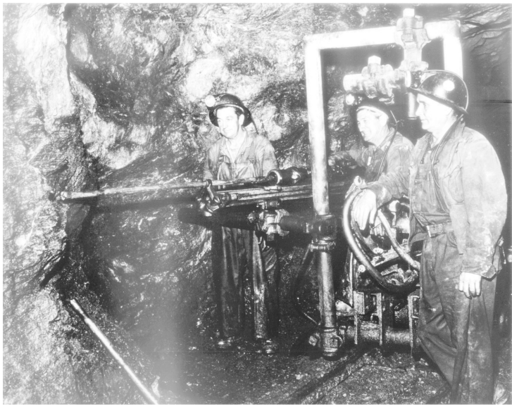
Miners drilling for ore
